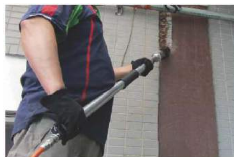
Corrosion removal for inaccessible area
